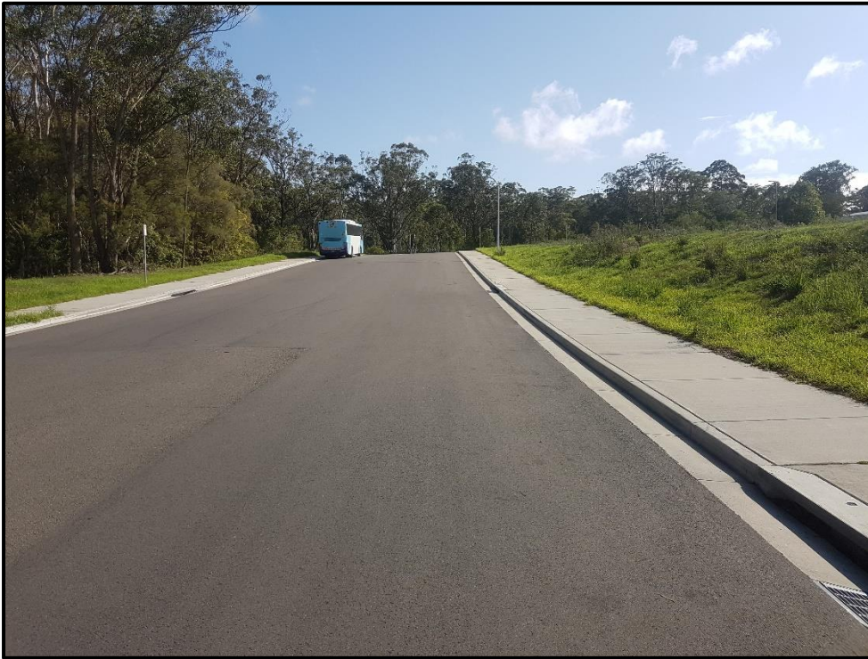
Photo 1 – Cross section of Peppertree Road looking north, subject site to the right
